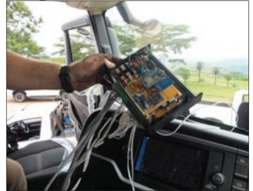
▲ The data logger in the cab was connected wirelessly to various input points.
